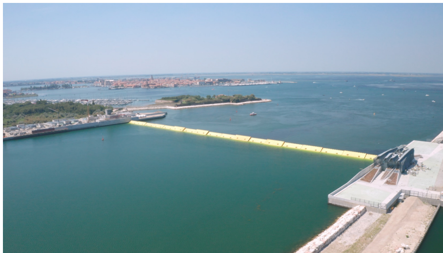
Figure 5 MOSE barrier closes the Lido inlet (S. Nicolò side), during a test (The original source of this figure is: Courtesy of Consorzio Venezia Nuova- Concessionary of Ministry of Infrastructure of Italy)
