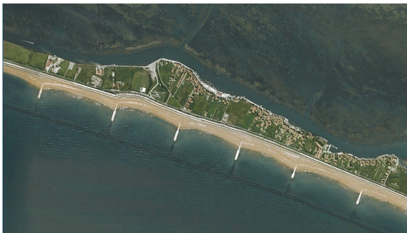
Figure 3 The new shore realized in front of the old “murazzi” in the Pellestrina island (The original source of this figure is: Courtesy of Consorzio Venezia Nuova- Concessionary of Ministry of Infrastructure of Italy)
