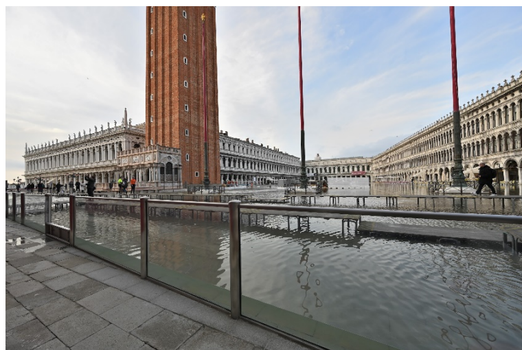
Figure 8 The glass barriers in front of St. Mark's Basilica provide effective protection also from minor "acqua alta" events
