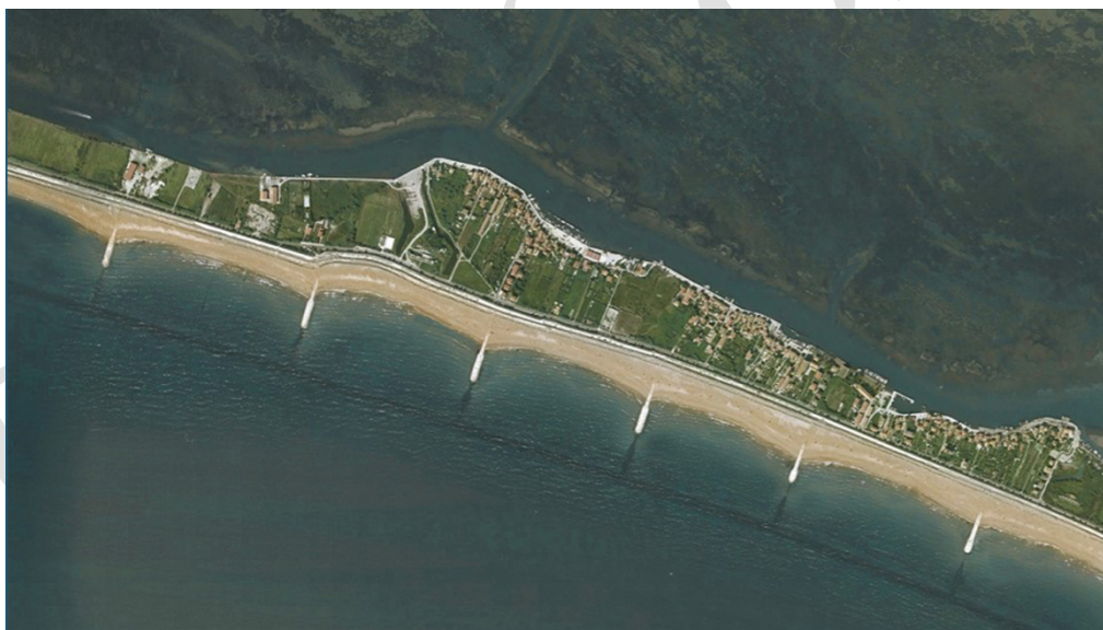
Figure 4. The new shore realised in front of the old murazzi on the island of Pellestrina. The original source of this figure is the Consorzio Venezia Nuova – Concessionaire of the Ministry of Infrastructure of Italy.
