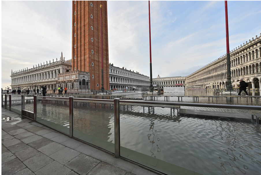
Figure 8. The glass barriers in front of St. Mark’s Basilica provide effective protection, also from minor “acqua alta” events.
