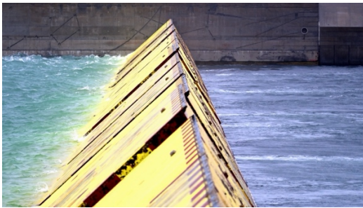
Figure 5 The MOSE barriers in Lido, during a storm, the 15/11/2020. In the picture, the sea on the left, the lagoon on the right. Figure 6 Sea level in the Adriatic (red) and inside the lagoon (blue) during the events of 3/10/2020 (left) and of 22/11/2022 (right)
