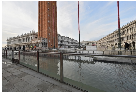
Figure 7 The glass barriers in front of St. Mark's Basilica provide effective protection also from minor “acqua alta” events
